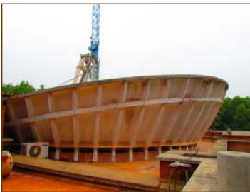
Largest Solar Kitchen in South Asia at Auroville, India Solar collector is made with ferrocement.
